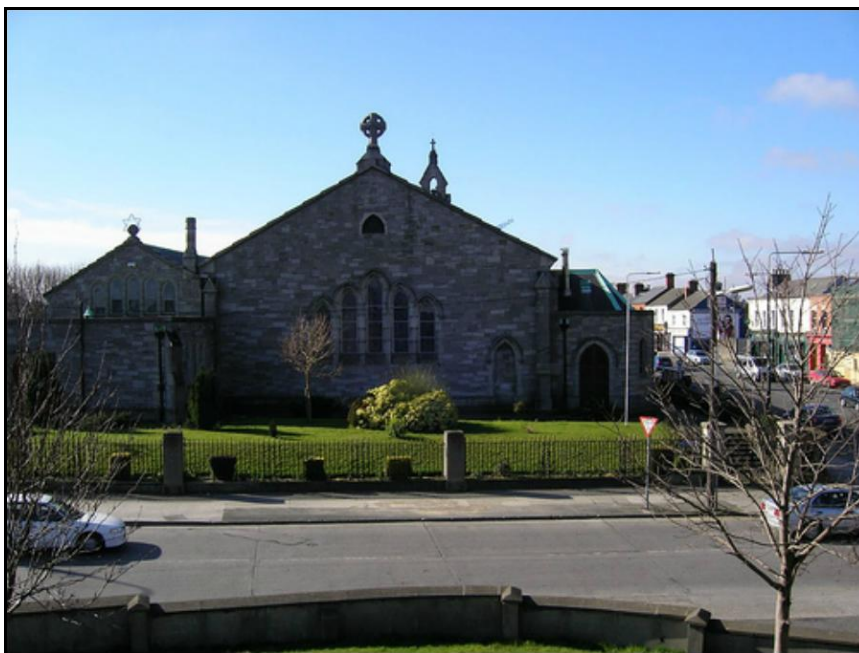
Figure 11: St. Michaels Church (view from Bulfin Road)
