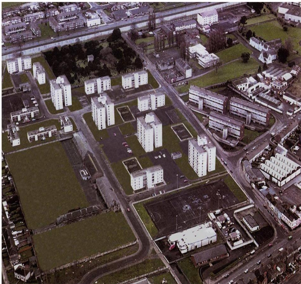
Figure 1: Aerial Photo of former St. Michaels Estate
