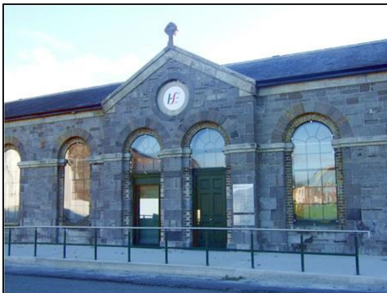
Figure 12: HSE Primary Health Care Centre
